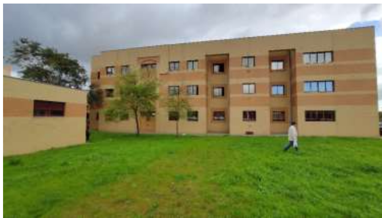
Figure 17. Lateral view of the building. Photo taken in March 4, 2020.
