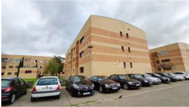
Figure 18. Frontal view of the building. Photo taken in March 4, 2020.
