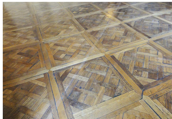
Figura 0.2: Parquet (Builddirect - Hardwood flooring history, 2020)
