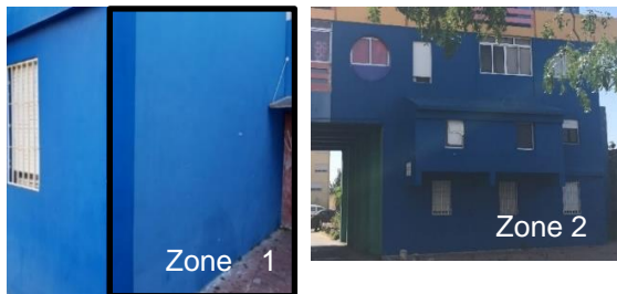
Figure 1 - Thermal render applied in 2014 (Zone 1) and in 2015 (Zone 2)
