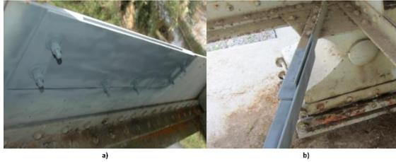
**Figure 4:** Places of sampling: (a) lower truss rope core plate; (b) diagonal of lower bracing near the right abutment [25].
