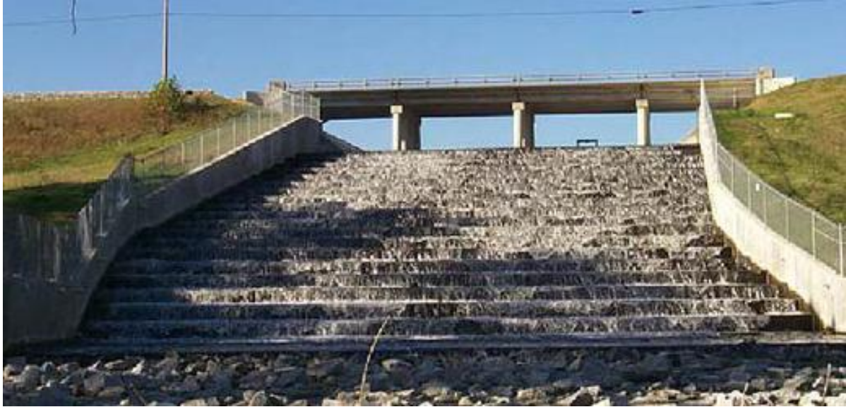
Figure 2.5: Stepped spillway in Stone Mountain dam, Georgia, USA [16]
