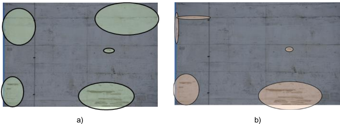
Figure 6 –Identification of critical using the SC-Anom results (a) and the visual detection results (b);
