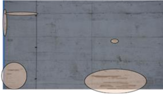
Figure 3 - Identification of critical zones in panel 13;
