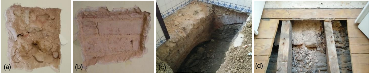
Figure 4 Viewing windows carried out: (a) JI 3 - Irregular stone masonry; (b) JI 13 - Brick masonry; (c) Probing well (PS); (d) Wood floor (IP B)
