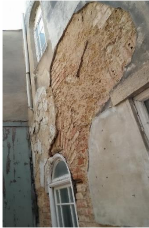
Figure 5 Masonry arch over window (orange)
