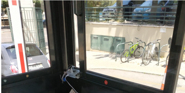
(a) TR Evo Installation
