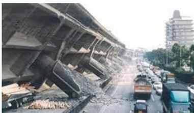
**Figure 1.1**-Collapse of the Hashin expressway due to Kobe earthquake (1995) [1].
