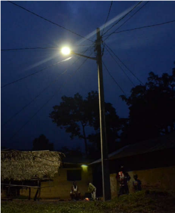
Figure 6.7: Outdoor Street Light
