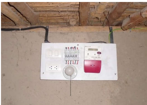
Figure 6.4: Household Electric Board
