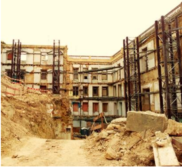
Figure 2 – Façade stabilization structure.
