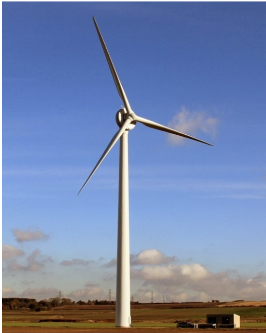
(a) Horizontal Axis Wind Turbine (HAWT)
