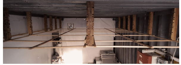
Figure 5: Final wooden structure without PCM boards.
