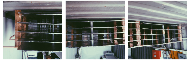
(a) Wooden structure with PCM boards (1/3). (b) Wooden structure with PCM boards (2/3). (c) Wooden structure with PCM boards (3/3).
