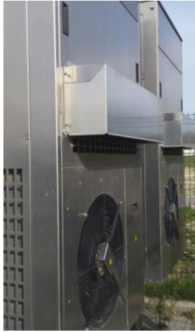
Figure 3-3: Cooling units: large container setup with 2 x PTAC units (left), small container setup with 1 x PTAC and 1 x Split unit (right)
