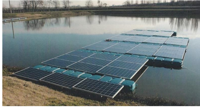
Figure 24: Example of floating platform built with cubic buoys [39].
