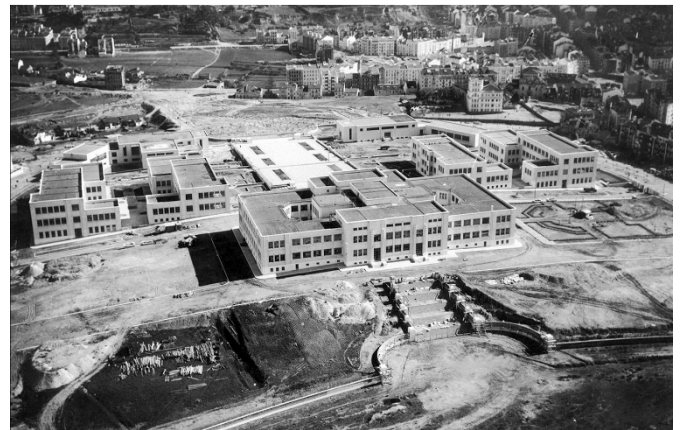
Figure 1: Aerial photograph of the Instituto Superior Técnico circa 1934
