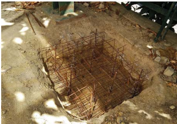
(a) Steel cage.
