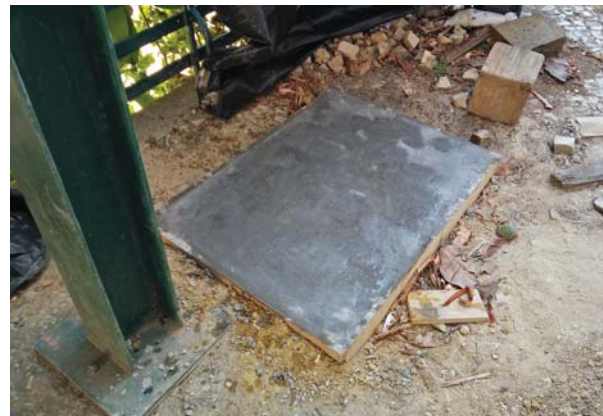
(b) Finished reinforced concrete block.
