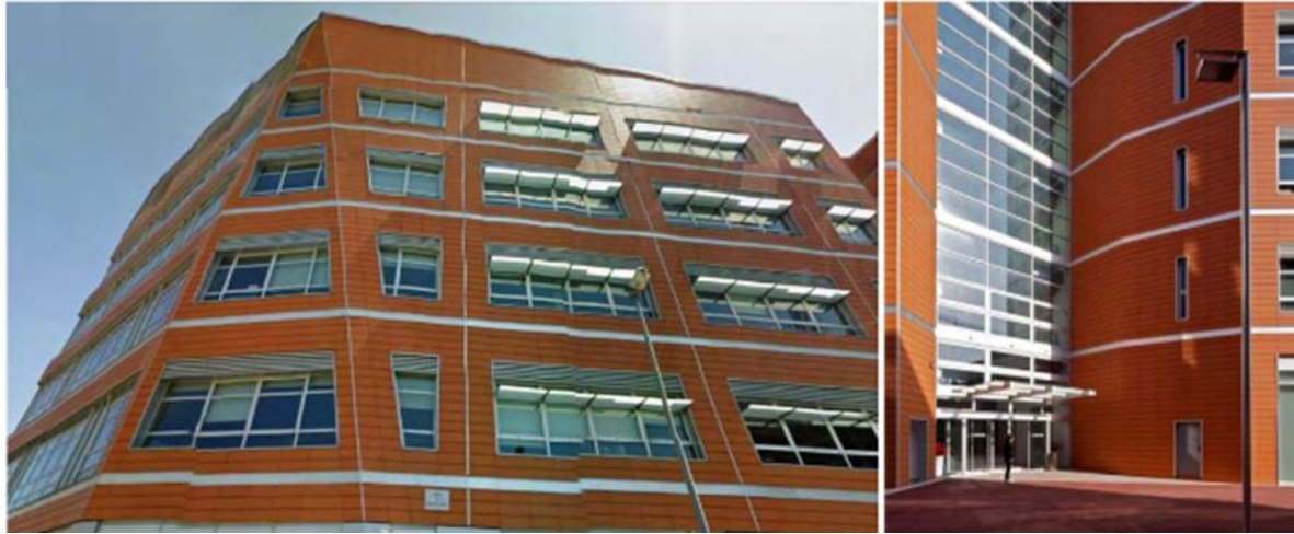
Figure 13 Shades on the façade on the left and entrance with the atrium on the right in ICAEN
