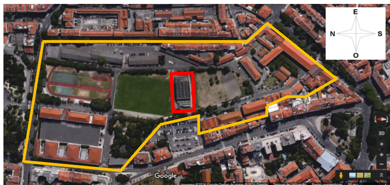
Figure 3.1 – Location of the indoor pool of the Military Academy (Satellite image taken from Google Maps, September 15, 2016)
