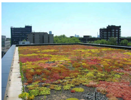
Figura 2.9 - Exemplo de um “ Extensive Green Roof ” (Environmental Department of Düsseldorf, 2009).
