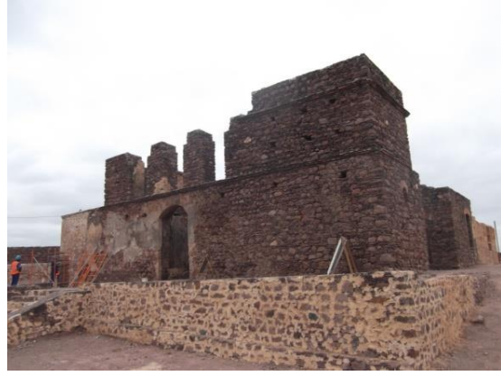
Figure 2 – Main facade walls.
