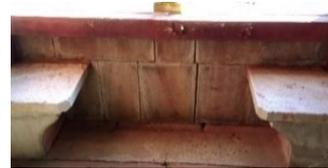
Figure 14 - Non-functional joints of a window framing
