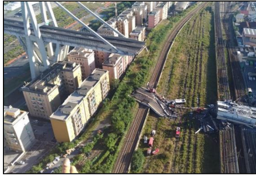
Figure 1.1- Aftermath of the Morandi Bridge collapse
