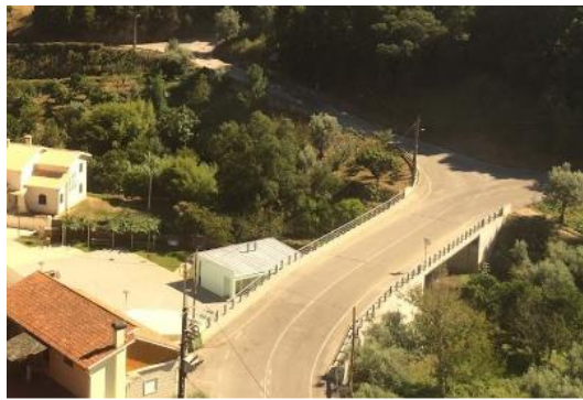
Figure 4.1- Aerial picture of the Várzeas Bridge
