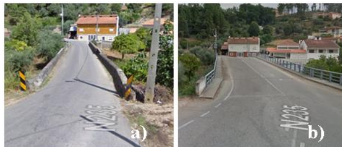
Figure 4.2- Road network on the site of the Várzeas Bridge a) before construction; b) after construction
