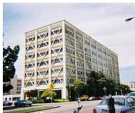
Figure 9 - Example of steel bracing on the exterior of a building (adapted from [14])
