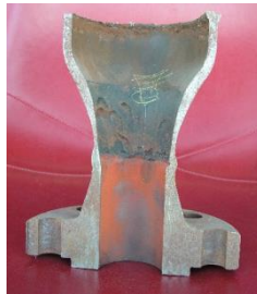
Fig. 5 - Erosion corrosion in the middle of a reducer [27].
