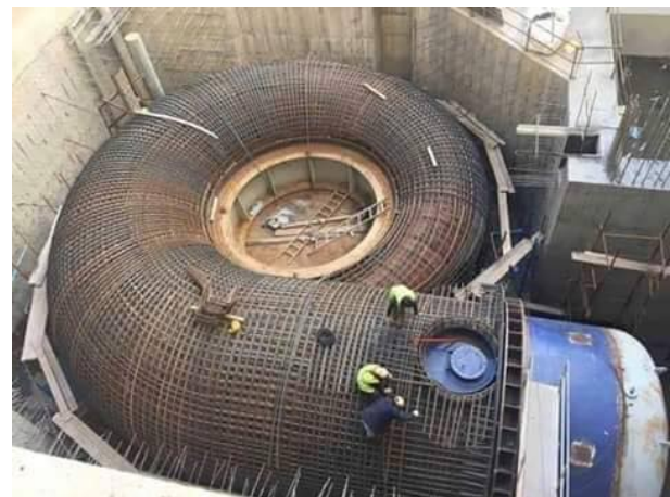
Figure 1.2: Example of reinforcement assembling surrounding spiral case for later concreting [10]
