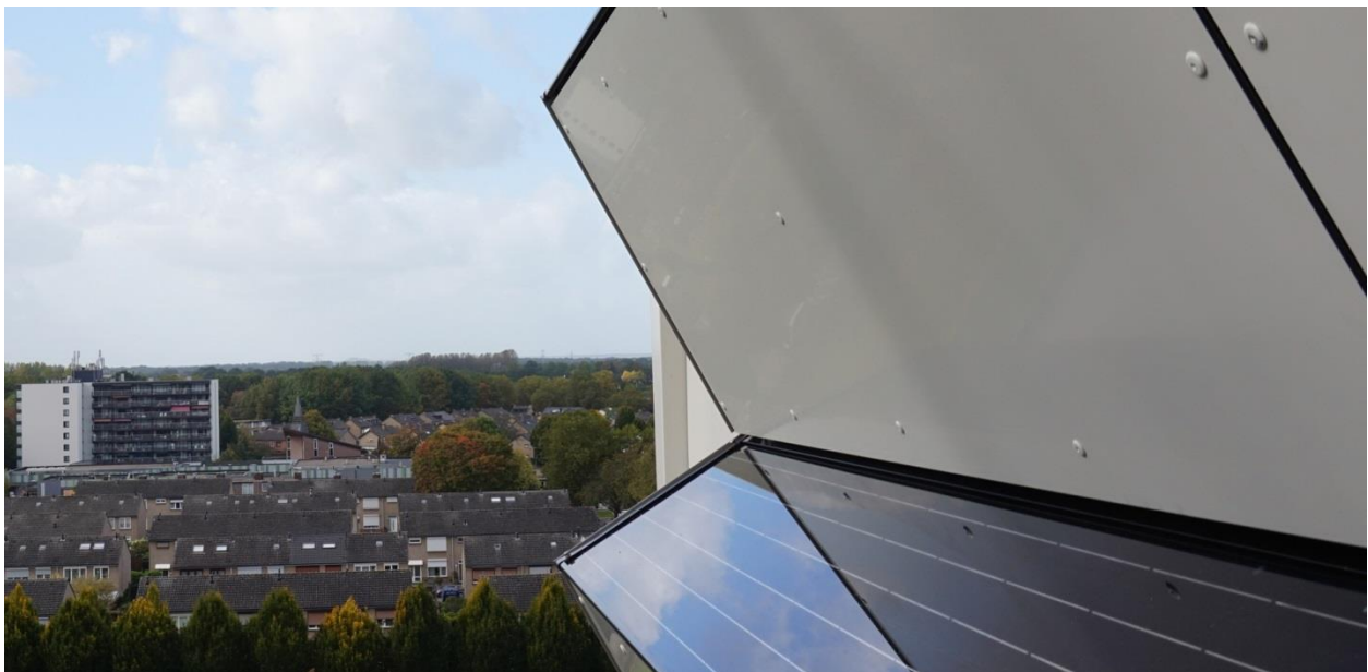
Figure 3.1: Eisenhower cassette showing the position of 1 module and reflector [40]
