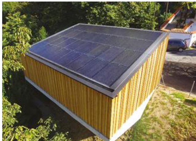
Figure 2.10 Prefabricated BIPV roof system [21]
