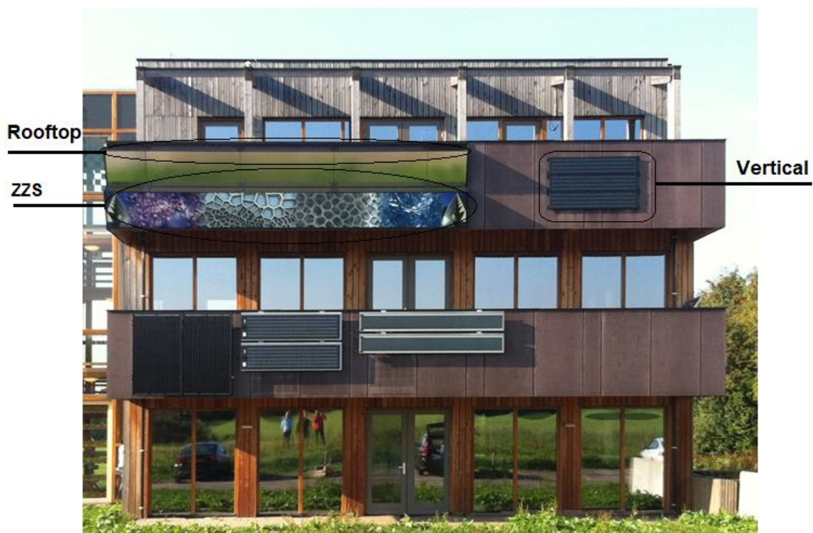
Figure 4.6: Wajk van Morgen ZVS, rooftop and vertical BIPV system [adapted from 40]
