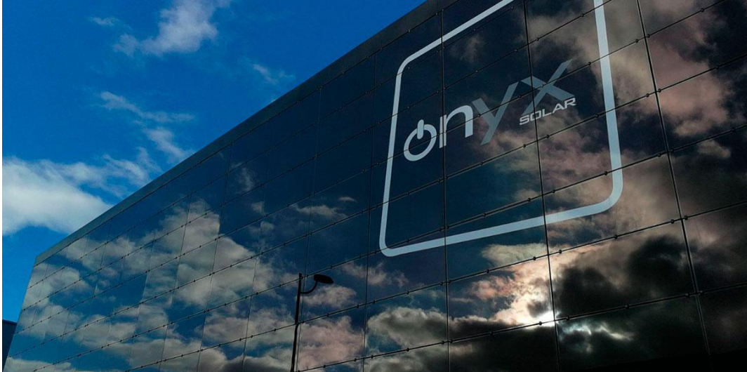
Figure 2.13 BIPV curtain wall [29]
