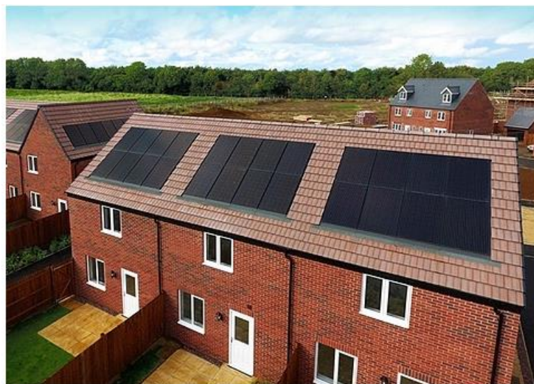
Figure 2.8 In roof BIPV system [25]
