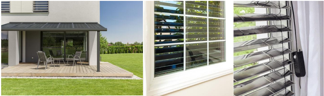
Figure 2.15 Canopy BIPV on the left [32]. Window blinds BIPV on the right [33]
