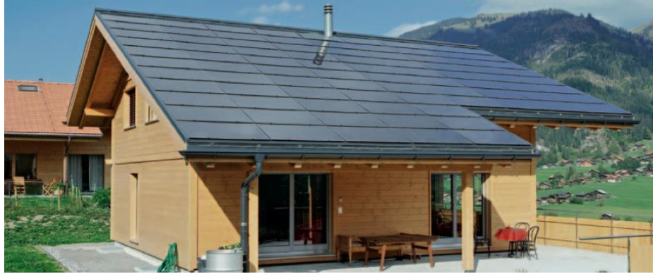
Figure 2.9 Full-roof BIPV system [26]
