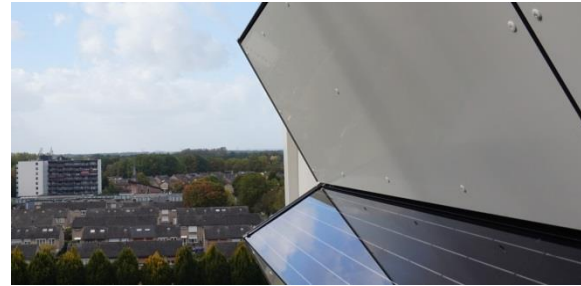
Figure 1: Eisenhower cassette showing the position of 1 module and reflector
