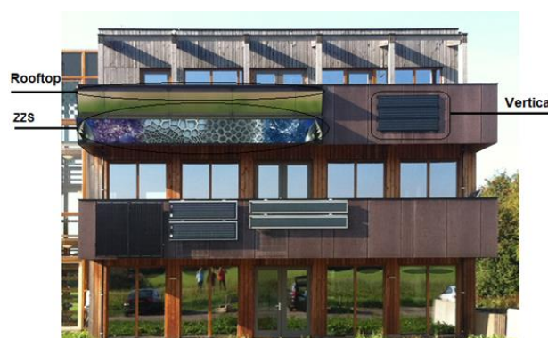
Figure 8: Wajk van Morgen ZSS rooftop and vertical BIPV system
