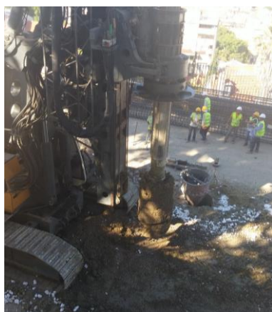
Figure 29 - Pile walls excavation (drilling machine)
