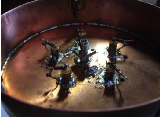
Fig. 11 - Electrical components associated with monopoles
