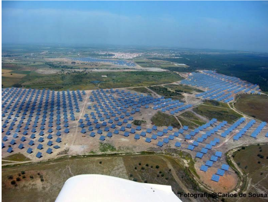
Figure 1-12: Amareleja (Portugal) PV power plant. Source: http://geoelvas.blogspot.pt/2013/08/central-solar-fotovoltaica-de-amareleja.html
