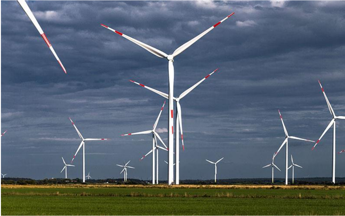
Figure 1-3: Onshore wind park; Source: . https://www.power-technology.com/projects/galway-wind-park/
