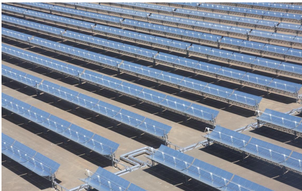
Figure 6-3: Parabolic trough power plant; Source: https://www.sbp.de/en/project/parabolic-trough-power-plant-andasol-ii/ .
