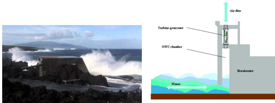
Figure 3.3: The Pico Power Plant (concluded in 1999, decommissioned in 2018), an onshore Wave Energy Converter of the Oscillating Water Column (OWC) type (source: left, WavEC; right, DOI 10.3390/en1112939). In an OWC, the heaving movement of the water inside a chamber compresses and expands the air, which can flow in and out the chamber through a turbine designed to always rotate in the same direction irrespective of the sense of the flow. The turbine drives a usual rotational generator.
