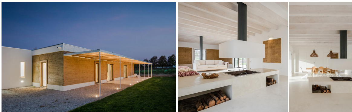
Figure 26 - Exterior and interior views of the Casa da Vinha in Montijo (source: blaanc, 2022)
