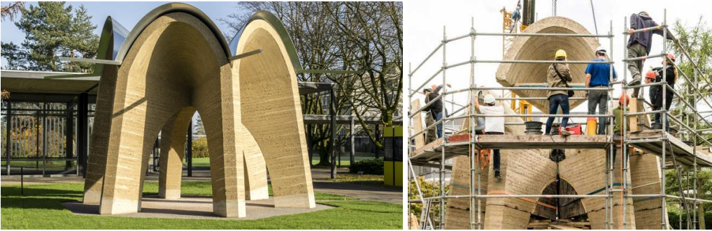
Figure 4 - Rammed earth vault (source: ETH, 2014)
