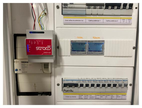
Figure 3.21: Smart meter solution in the electrical panel
