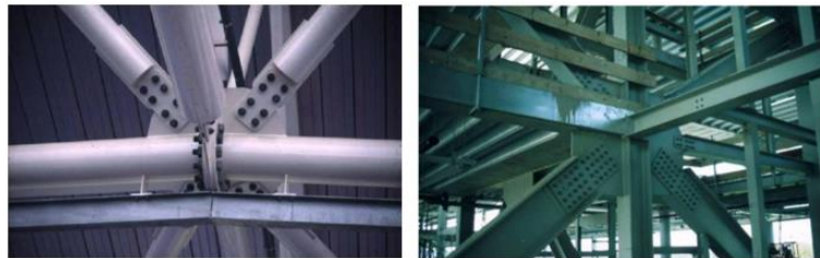
Figure 2.1: Structural hollow section joints.
