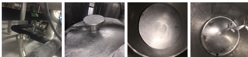
Figure 3.3: Sampling locations for validation and monitoring of CIP in ageing tanks: Outlet for rinse medium (left, original photos), Tank vent from the outside and inside of the tank (centre, original photos), Inner surface of tank (right, original photo)
