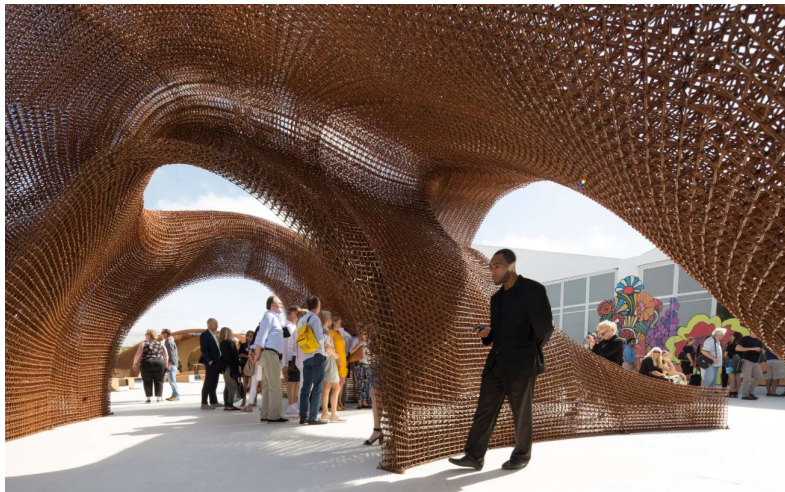
Figure 2.30: Pavilion made of 3D printed lattice structures [43]
