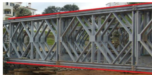
Figure 14 – Location of the chords strengthening (in red)
