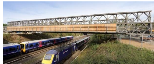
Figure 11 - Panel Overlapping on UK, adapted of Mabey Bridge 2020
