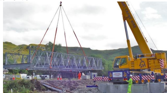
Figure 2 - Assembly using a crane, adapted from Mabey Bridge
