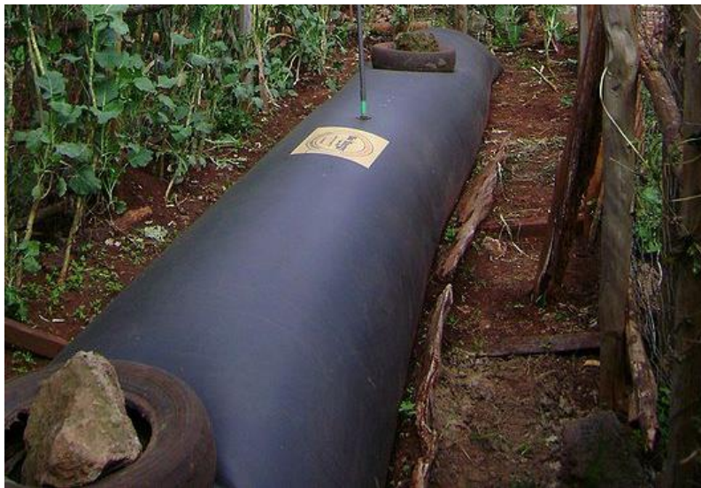
Fig. 2. 1 - Horizontal polyethylene-based tubular [56].
