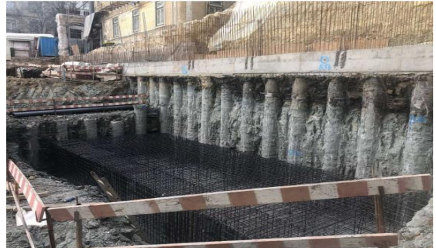
FIGURE 5 - FOOTING'S REINFORCEMENT
