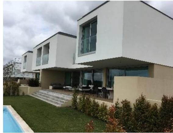
Figure 5 Townhouse 307 overview of terrace and swimming pool
