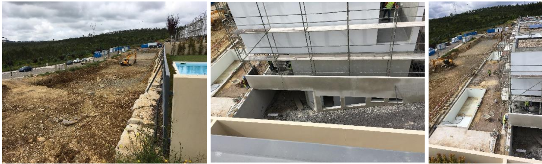
Figure 29 Townhouses construction process
