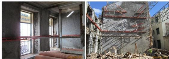
Figure 8- Photos of the demolition and façade retention processes.
