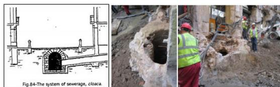
Figure 9 – System of sewerage, cloaca.
