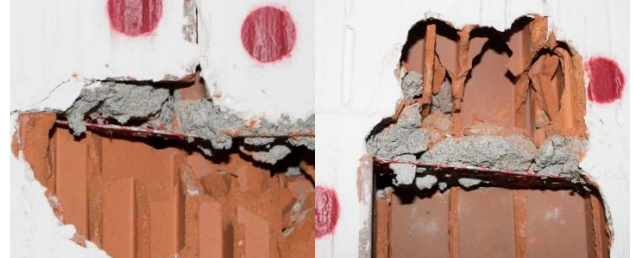
Fig. 15 – Murfor Compact I reinforced truss being solicited in tension.
