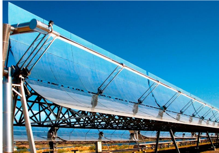
Figure 3 Concentrator with cylindrical trough collector
