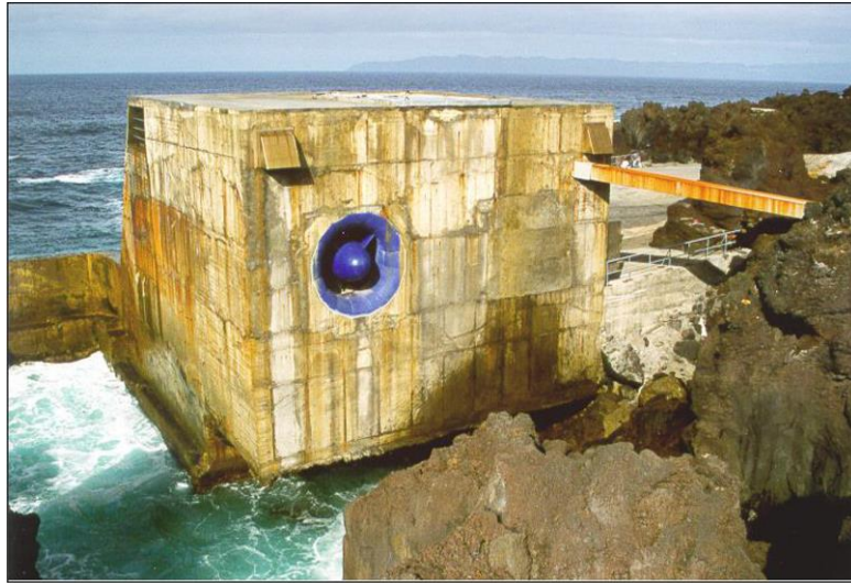
Figure 1: Pico plant, onshore OWC device, Azores, Portugal [4].
