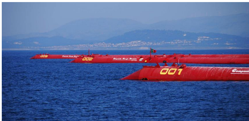
Figure 2: Pelamis plant, offshore floating devices with hydraulic PTO system, Aguçadoura, Portugal [1].
