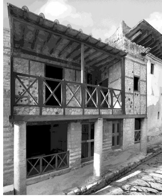
Figure 2-34 - The so-called Opus Craticium, an example of timber frame with masonry infill, in the ancient Roman town of Herculaneum, found after the archaeological excavations; Photograph by Randolph Langenbach
