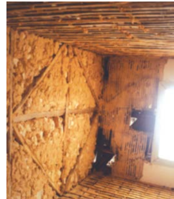
Figure 2-18 - Gaiola wall with the masonry filling
