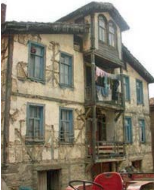
Figure 2-30 - Hatil at ground floor and himis in upper storeys (Turkey)
