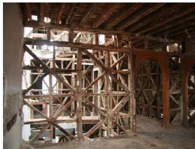
Figure 2-17 – Views of the Gaiola system after removal of cover and masonry, in a building recently demolished in downtown Lisbon
