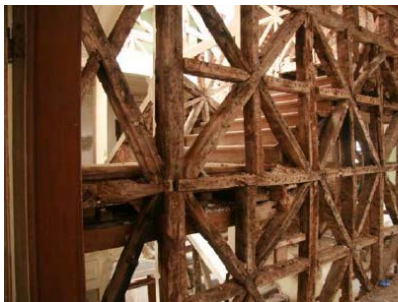
Figure 2-17 – Views of the Gaiola system after removal of cover and masonry, in a building recently demolished in downtown Lisbon
