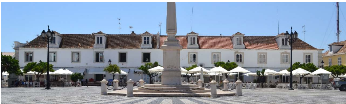
Figure 3-2 – Picture of the building during the on-site survey in VRSA
