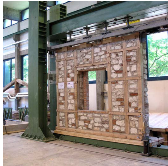
Figure 2-27 – Real scale model of the wall of Mileto Bishop's Palace, Laboratories of the Ivalsa CNR (Trento, Italy), 2013
