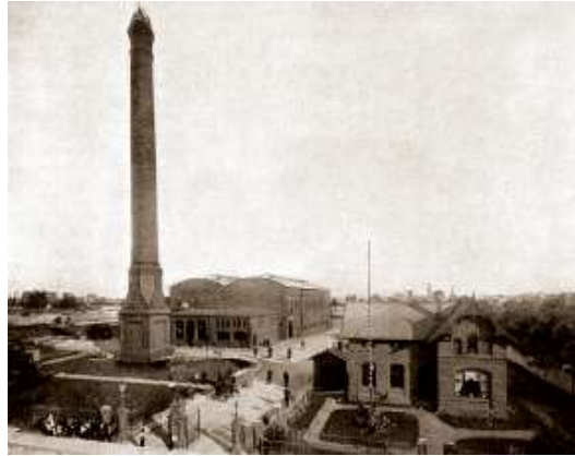
Figure 1. Incineration plant in Hamburg [2].
